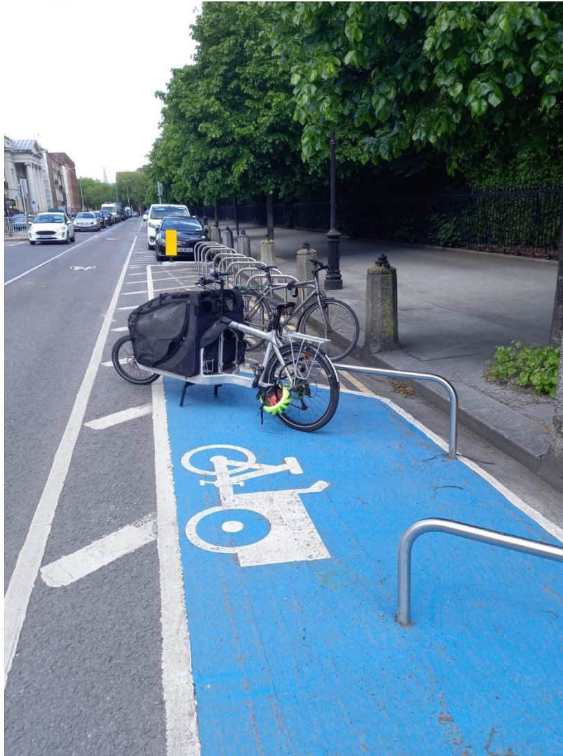
Figure 6. Example of short-term oversized bicycle parking in Dublin, which provides extra space for larger bikes and are delineated with paint to make it easier for users to find.
