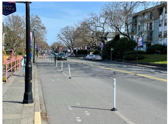
Adaptive Sidewalk on Oak Bay Avenue
