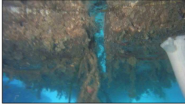
Figure 57 - Typical Marine Growth on Polystyrene Billets
