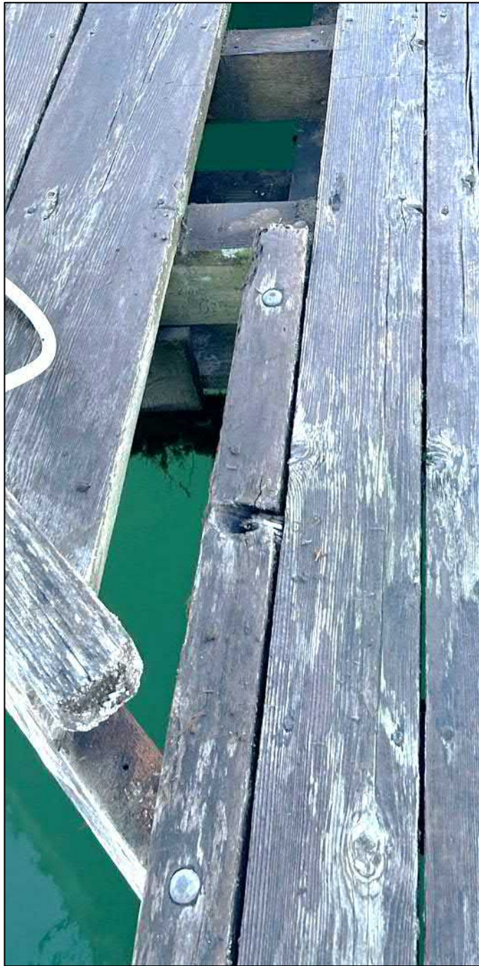
Figure 15 - Typical Configuration - Finger Connection to Wing Dock
