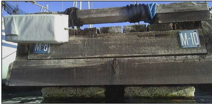
Figure 19 - Typical Configuration of Polystyrene Billets in Rows
