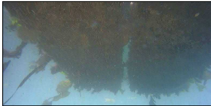
Figure 58 - Typical Marine Growth on Polystyrene Billets
