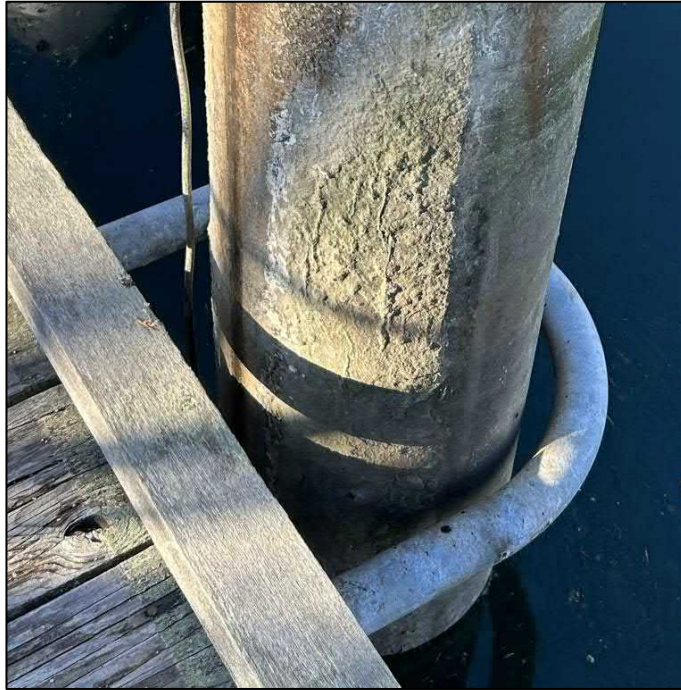
Figure 25 - Typical Pile Ring – Shown with a Steel Pile
