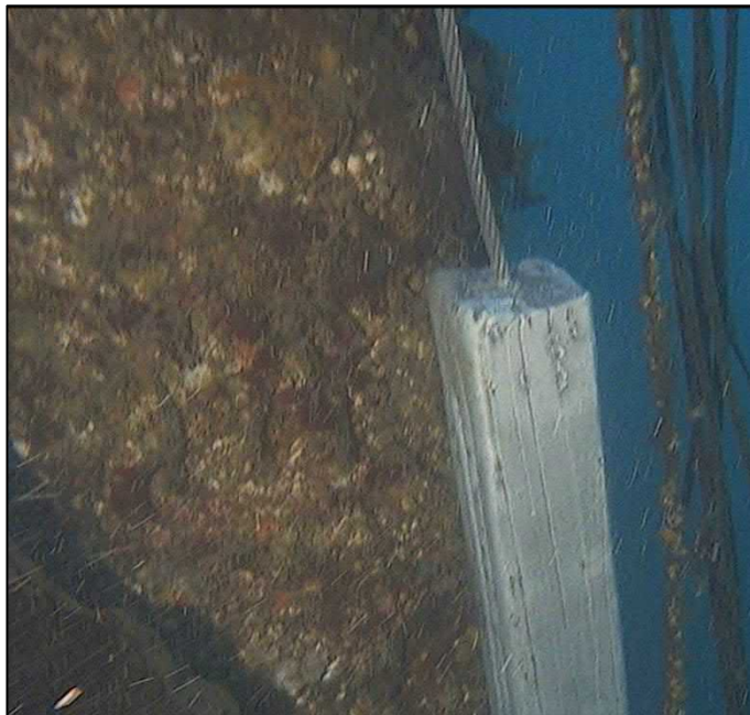
Figure 62 - Typical Galvanic Anode at Steel Pile
