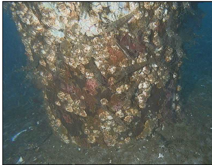
Figure 60 - Typical Base of Timber Pile
