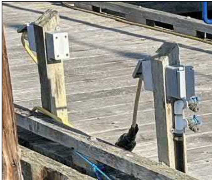
Figure 11 - Typical Configuration - Utility Post
