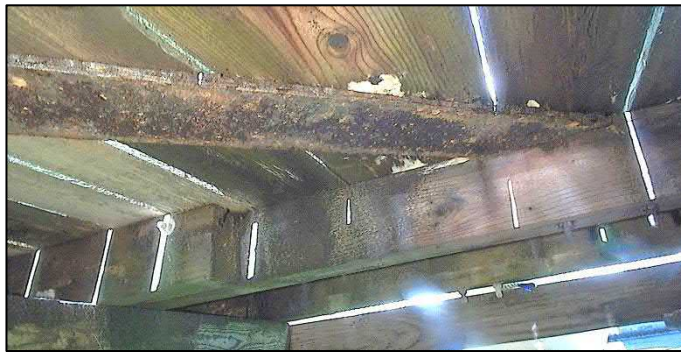
Figure 18 - Additional Steel Bracing at End of Dock G to Dock K
