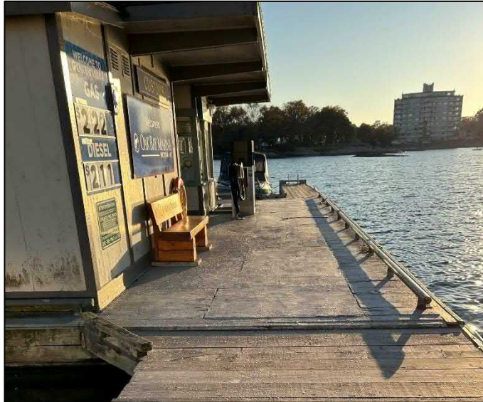
Figure 65 - Fuel Dock Topside View
