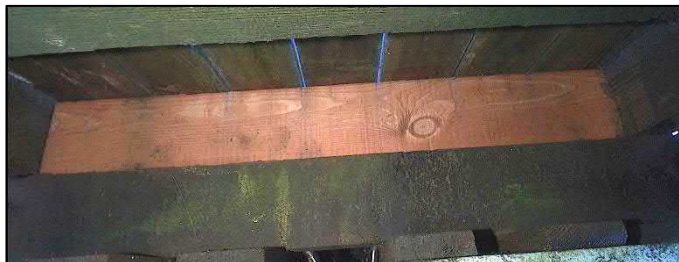
Figure 47 - Example of Framing Replacement
