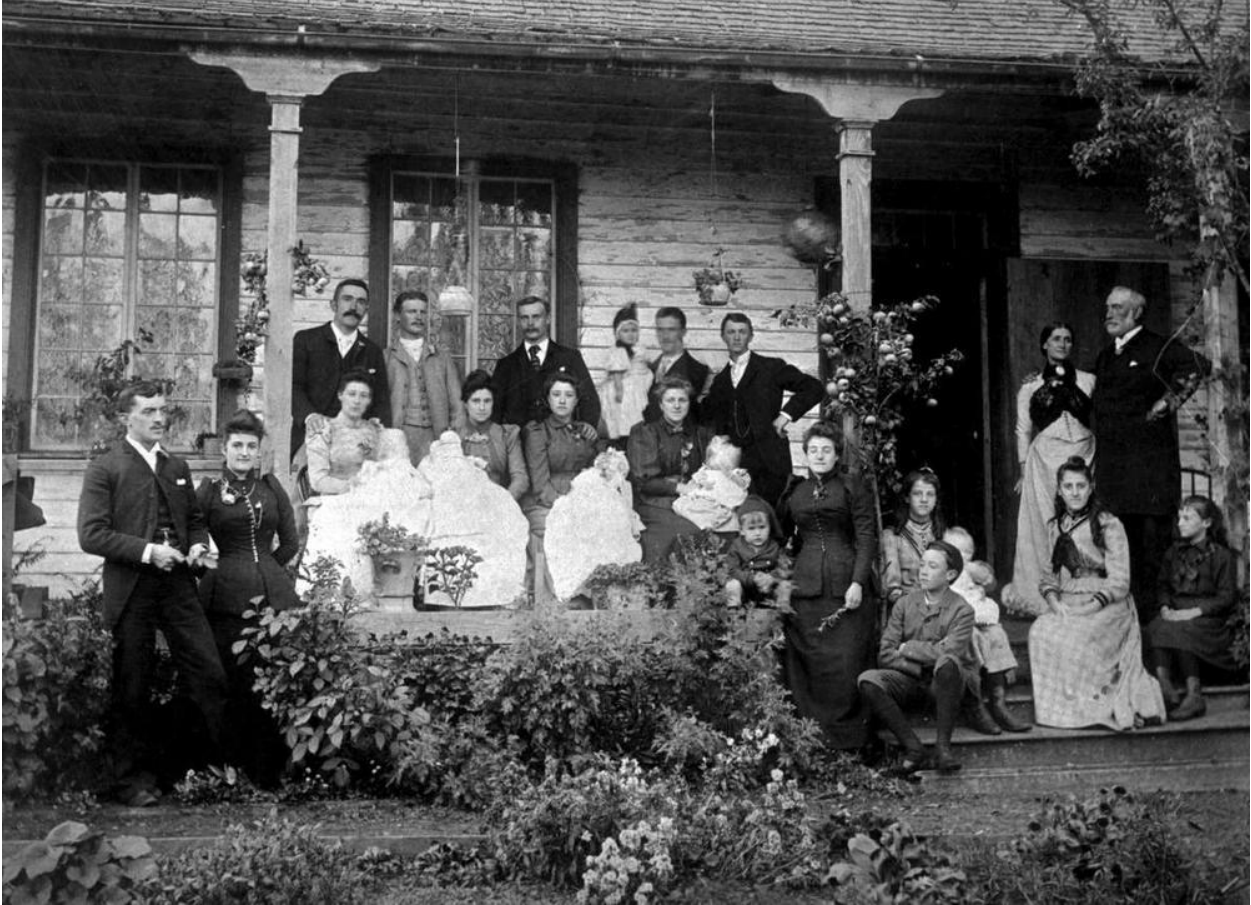
Figure 6 - Three generations of the Pauline family at Tod house in the 1890s. Note the wood posts and capitals, wood porch and steps, and plain transom light above the entrance door. J.K. Nesbitt collection. RBCMA A-08840
