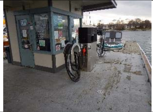
Photo 6 Description: Floating fuel dock
