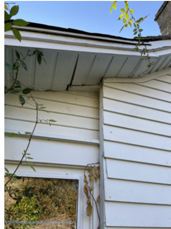
Soffit detail, North Elevation.
