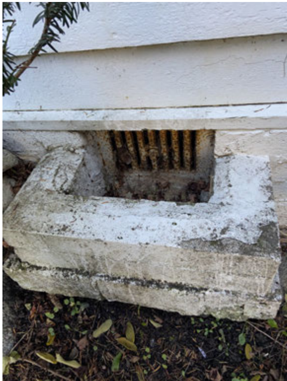
North Elevation. Vented crawl space.
