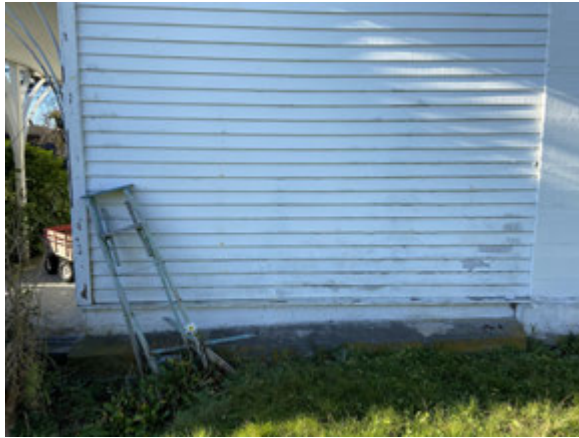
East Elevation, concrete curb poured against wall framing.
