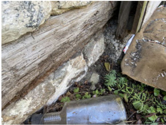
North Elevation. Original rubble foundation with hewn fir bottom sill.
