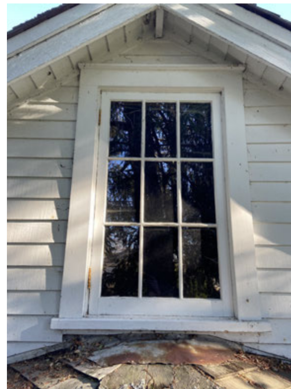
W12 Attic 1890s addition.
