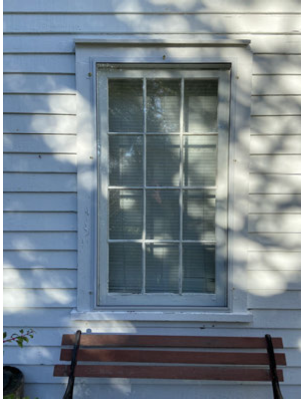
W13 South Elevation 1890s addition.
