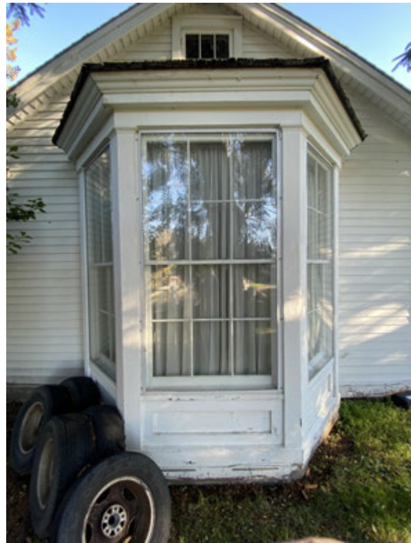
W10 Bay window 1890s addition.
