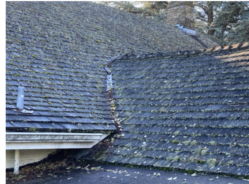
Typical roof valley.
