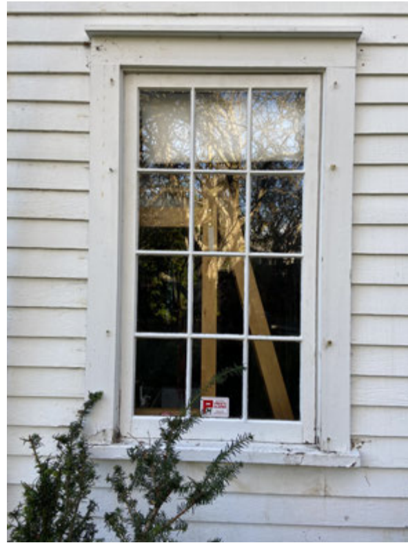
W7 North Elevation 1890s addition.
