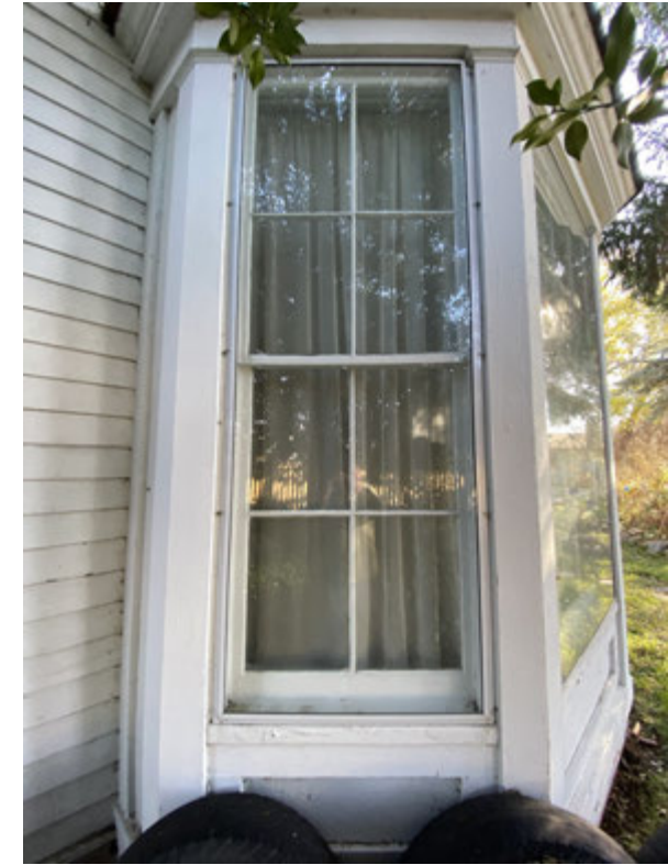
W9 Bay window 1890s addition.
