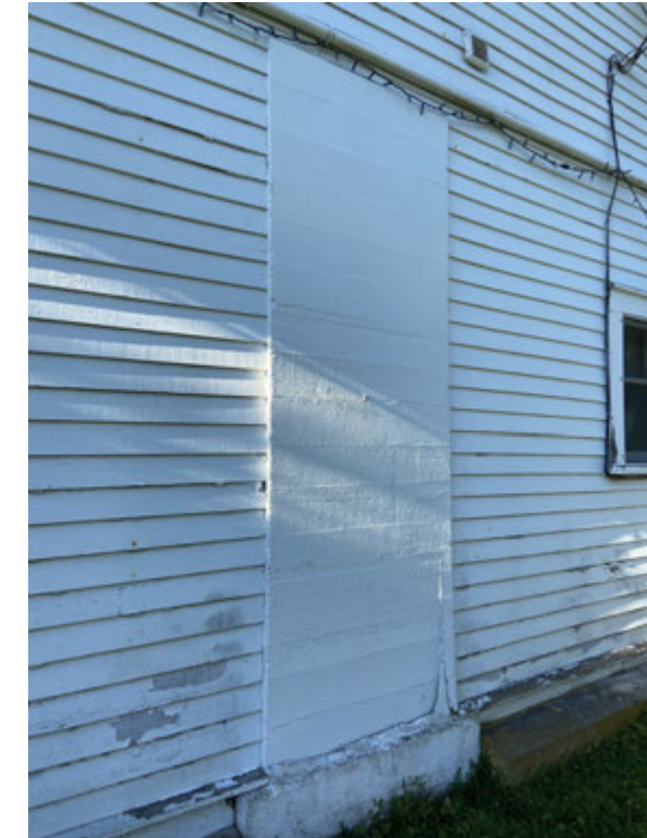
Brick chimney stack encased in concrete with form board finish to exterior wall .
