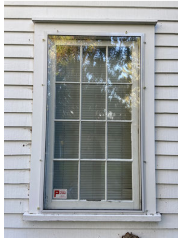
W8 North Elevation 1890s addition.
