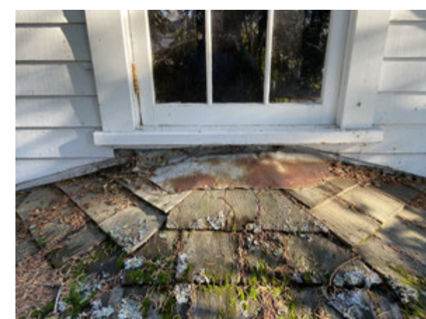
W12 sill with roof flashing.
