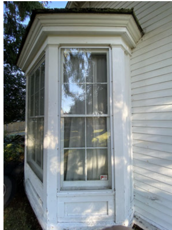
W11 Bay window 1890s addition.
