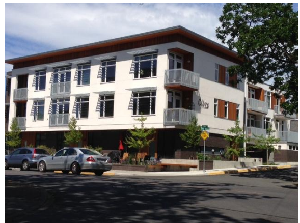
The Clive Project complete
