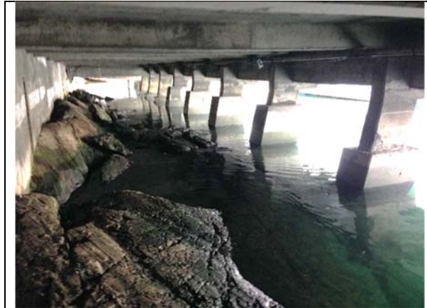
Figure 25-B: East-West concrete beams supporting building 25 offices.
