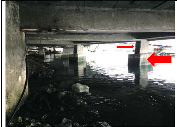
Figure 25-A: Radial beams supporting boardwalk and restaurant.
