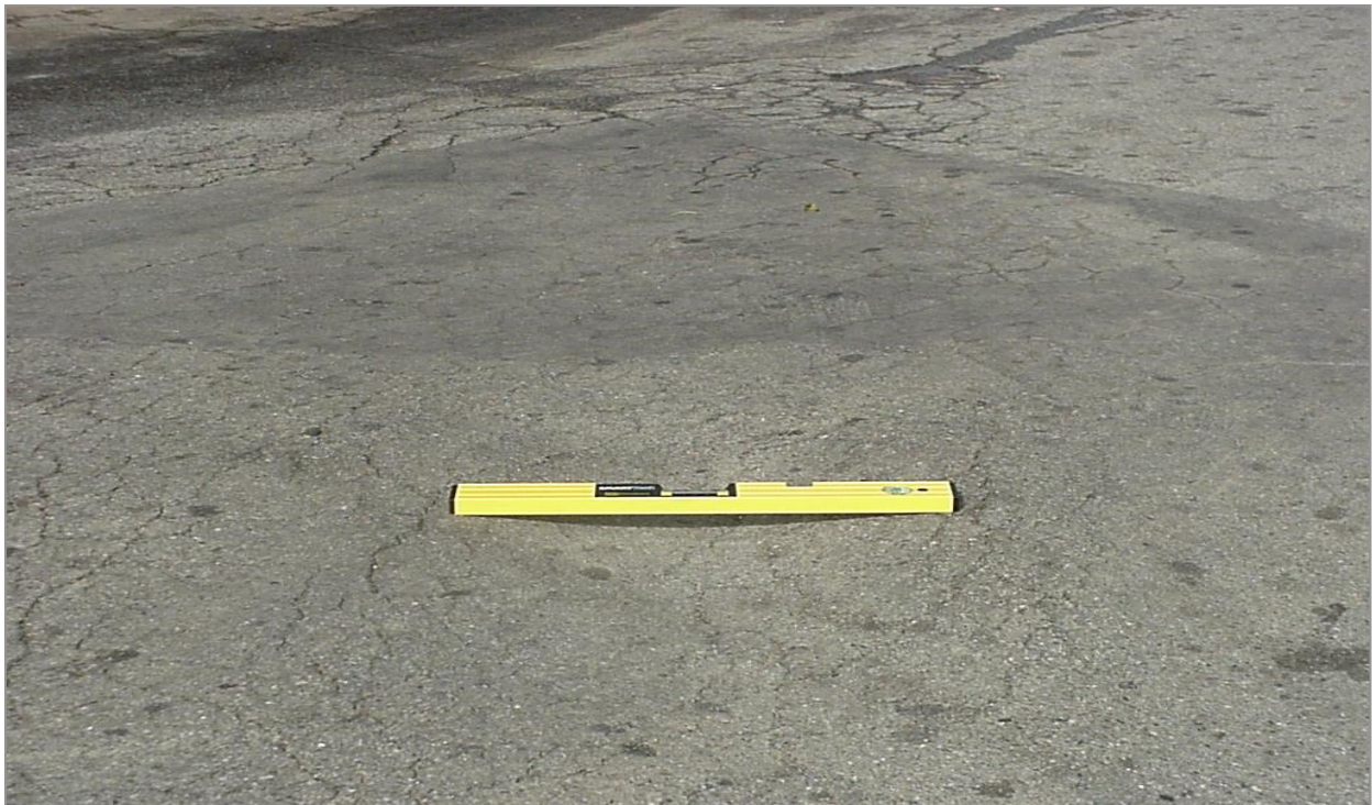
Figure 4.31: Slight Distortion (Image used for illustration)
