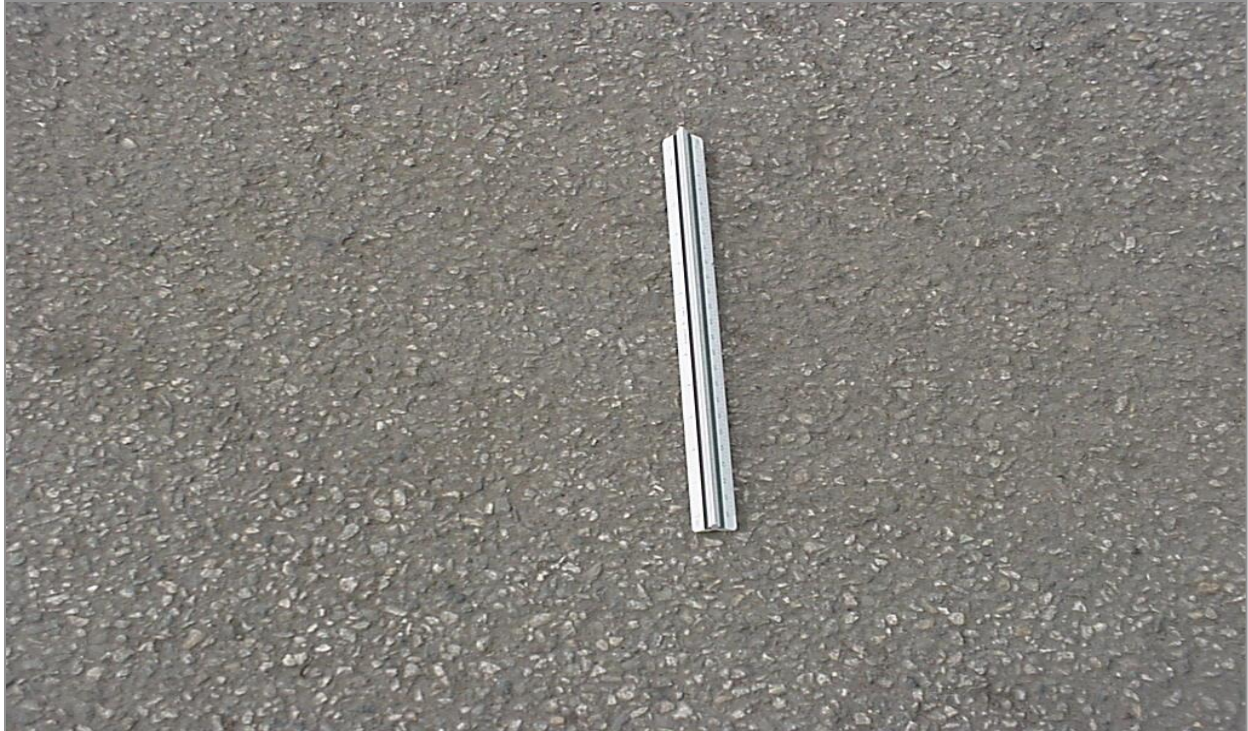
Figure 4.43: Slight Raveling (Image used for illustration)
