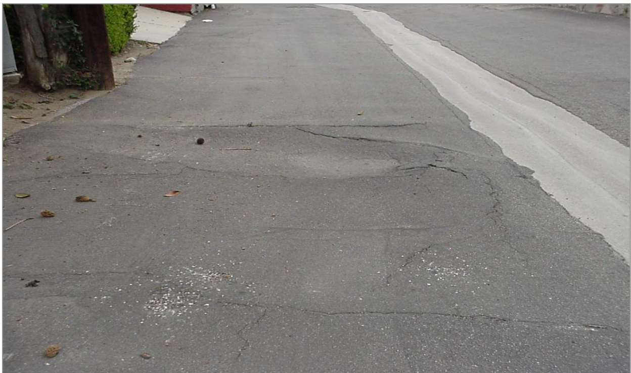
Figure 4.33: Severe Distortion (Image used for illustration)
