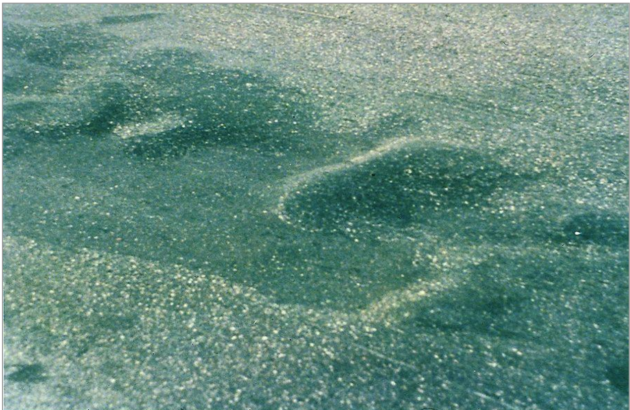
Figure 4.29: Severe Shoving (Rippling) (Image used for illustration)
