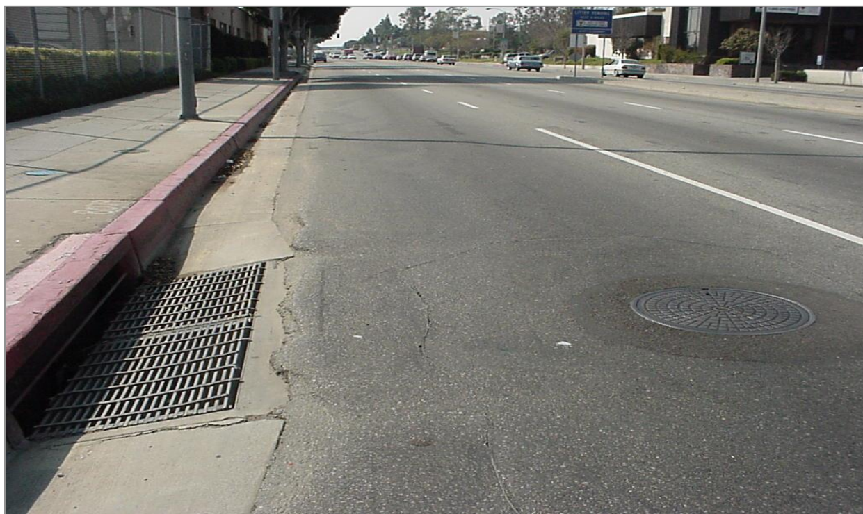
Figure 4.27: Slight Shoving (Rippling) (Image used for illustration)
