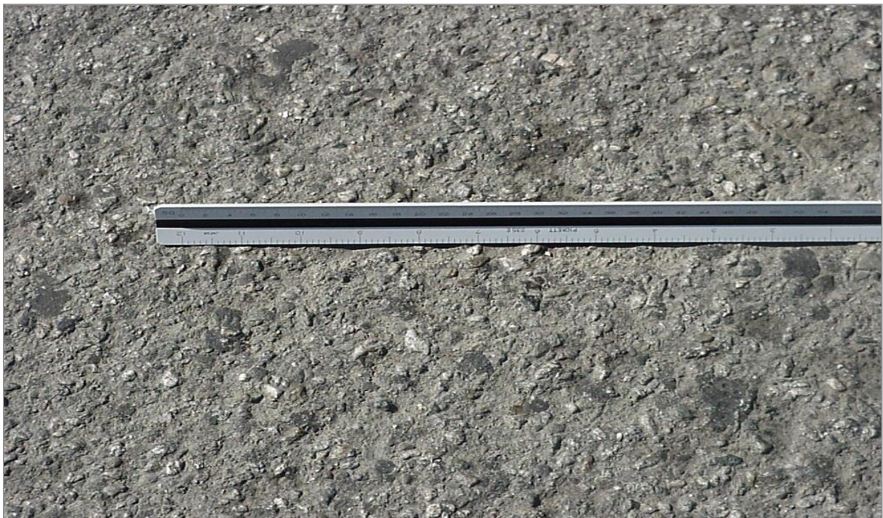
Figure 4.44: Moderate Raveling (Image used for illustration)
