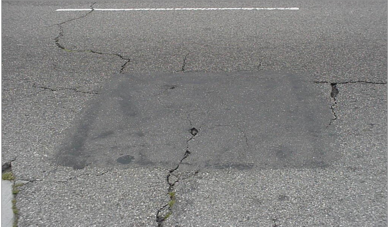
Figure 4.52: Moderate (Borderline) Patch (Image used for illustration)
