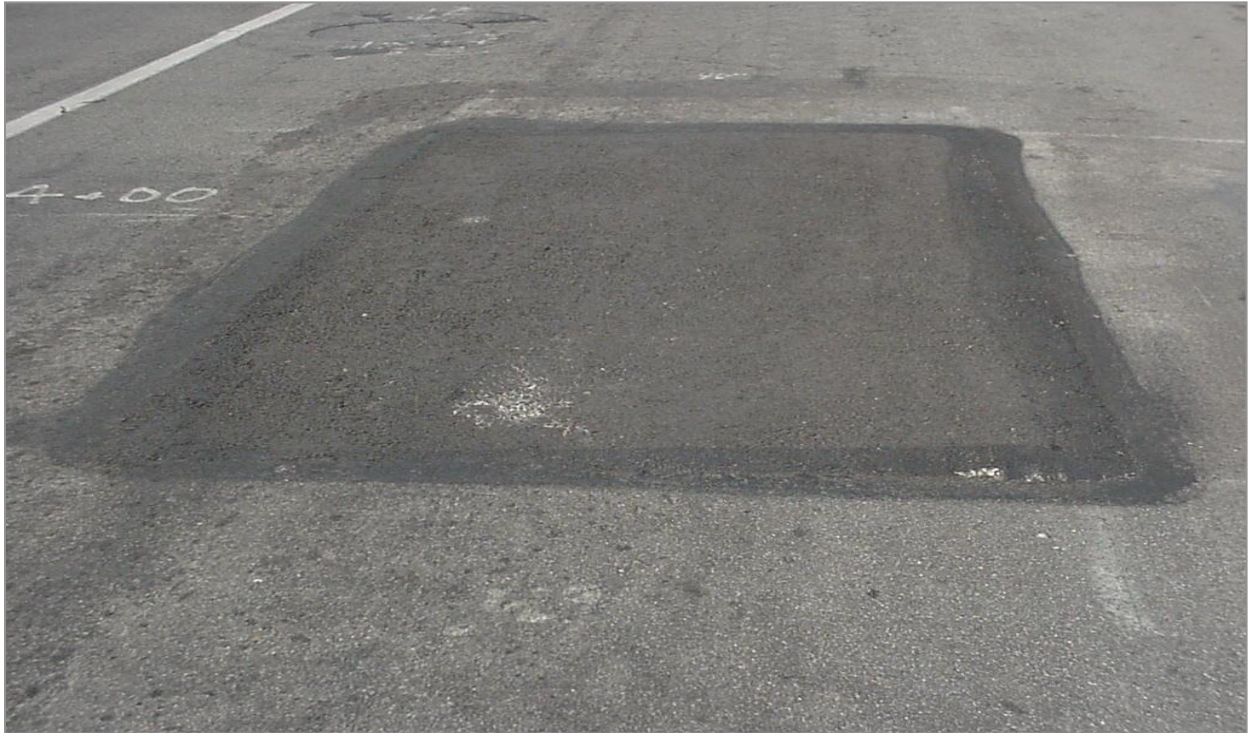
Figure 4.51: Slight (Good) Patch (Image used for illustration)
