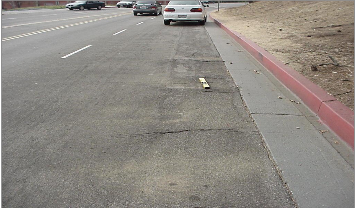
Figure 4.32: Moderate Distortion (Image used for illustration)
