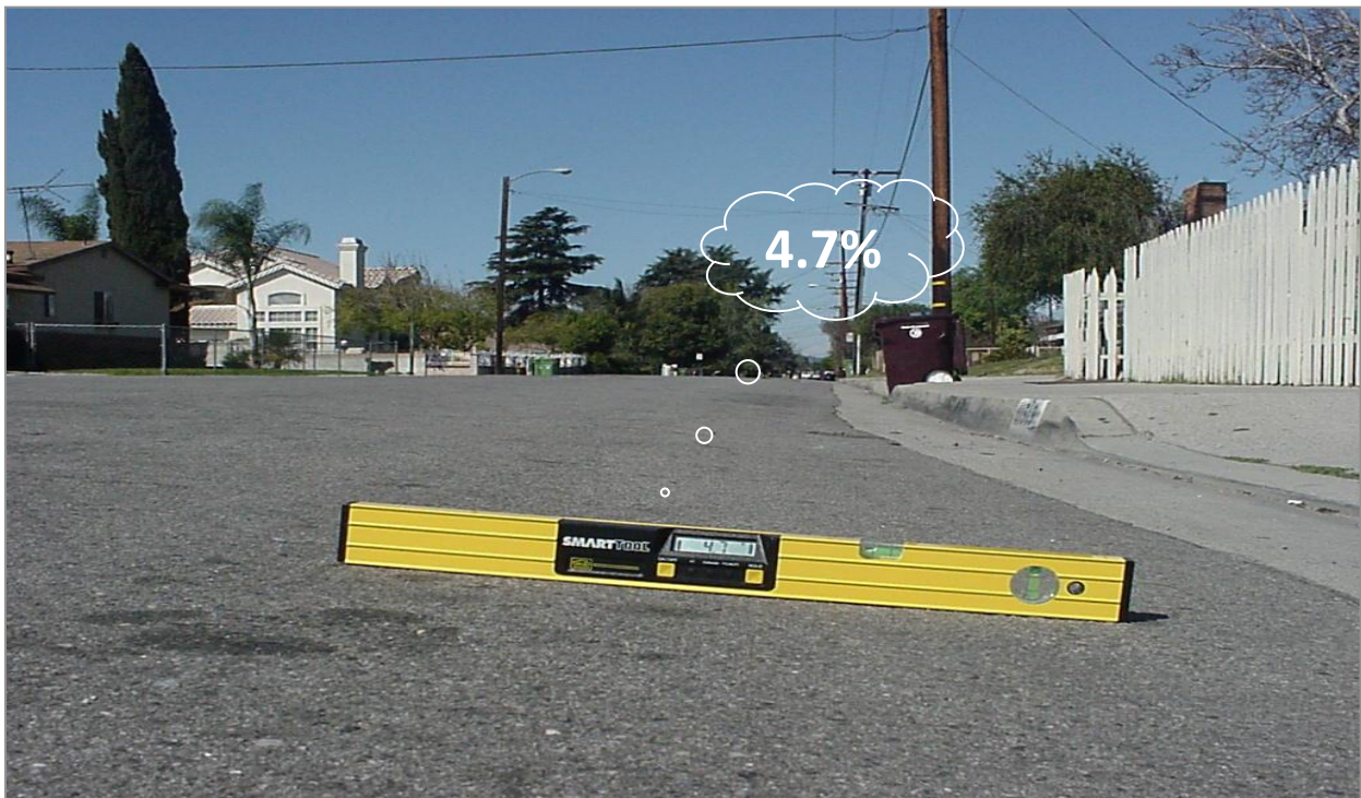
Figure 4.36: Moderate Excessive Crown (Image used for illustration)
