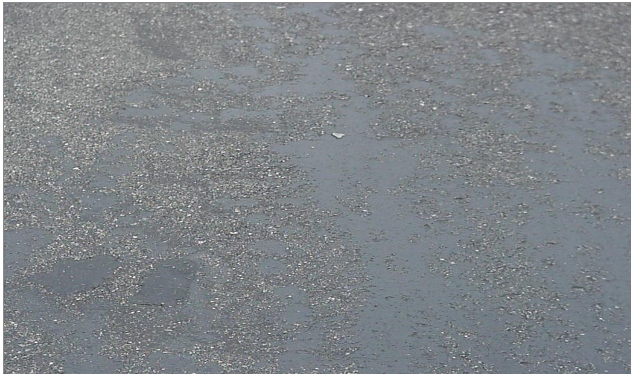
Figure 4.49: Severe Bleeding (Image used for illustration)
