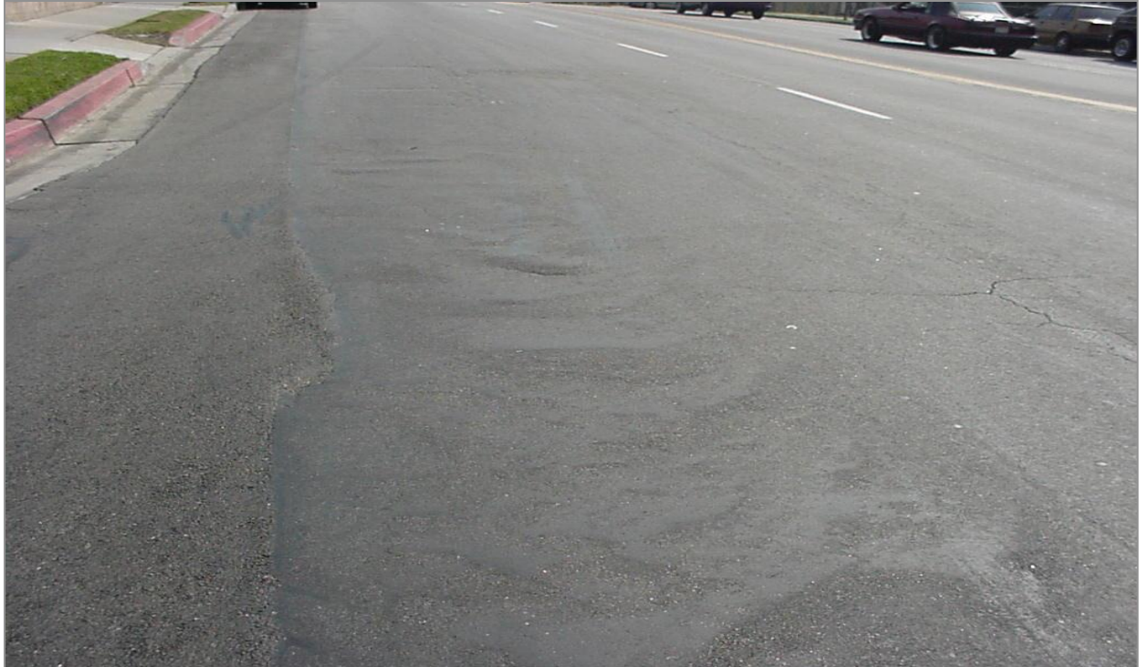
Figure 4.28: Moderate Shoving (Rippling) (Image used for illustration)
