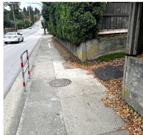
Example of a bed sted gate (Image credit: City of Coquitlam)
