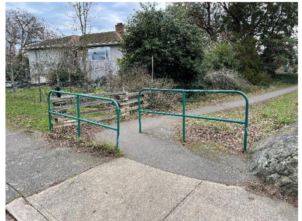
Example of a maze gate at Kings Road and Haultain Avenue
