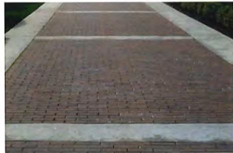
Roman pavers with concrete boarder
