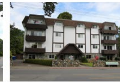
ADJACENT EAST PROPERTY FROM OAK BAY AVENUE
