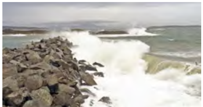
Turkey Head breakwater and perimeter riprap
