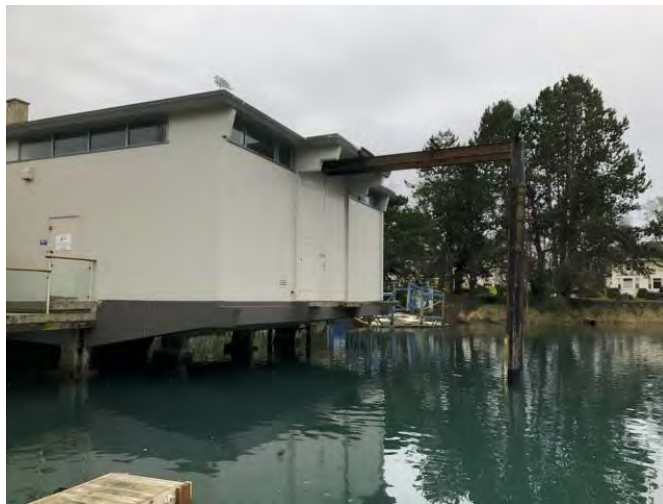
Photo #41: Dockworks West Elevation.
