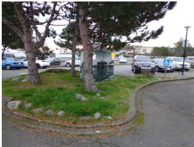
Photo #75: Site Light Posts Typical Landscaping and Transformer
