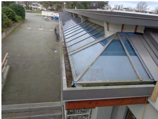
Photo #33: Office Skylight Canopy
