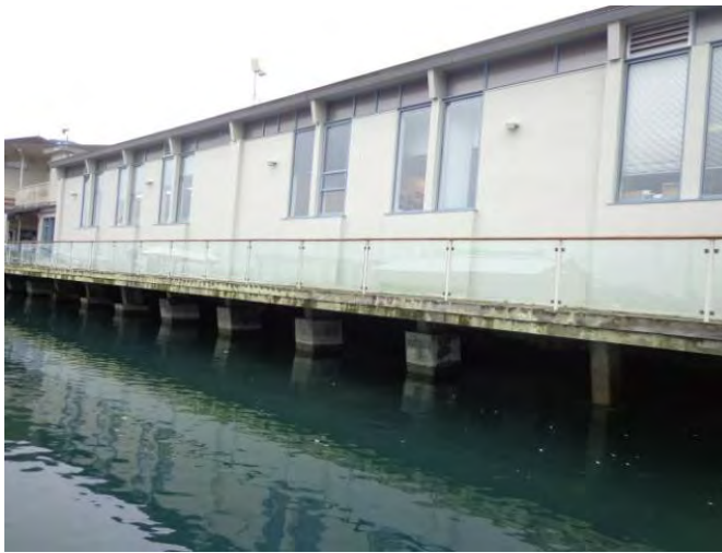
Photo #29: Office West Elevation
