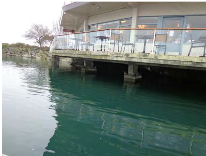
Photo #5: Restaurant Concrete Piles - Typical
