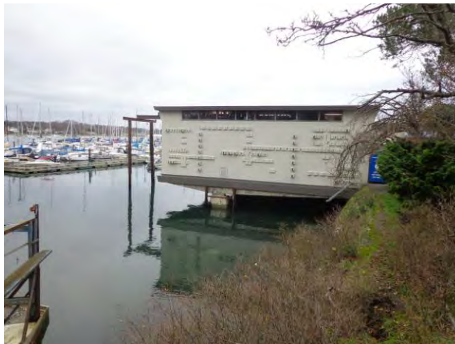
Photo #39: Dockworks South Elevation
