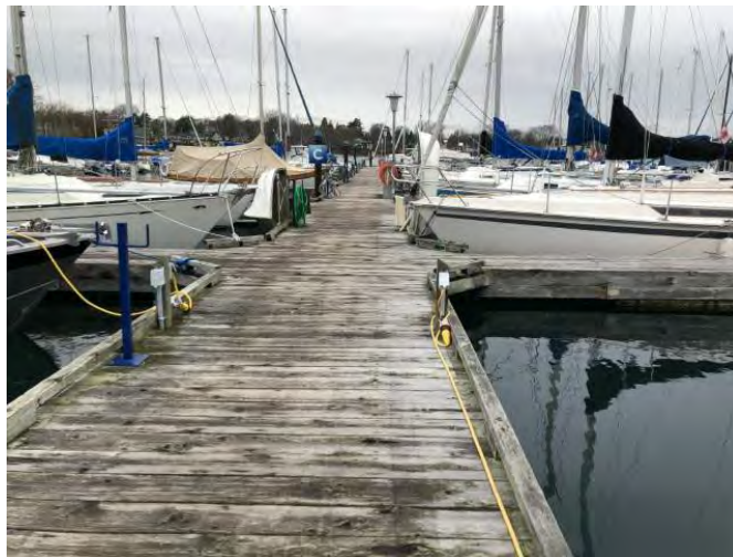
Photo #47: Marina Dock Walkways - Typical.
