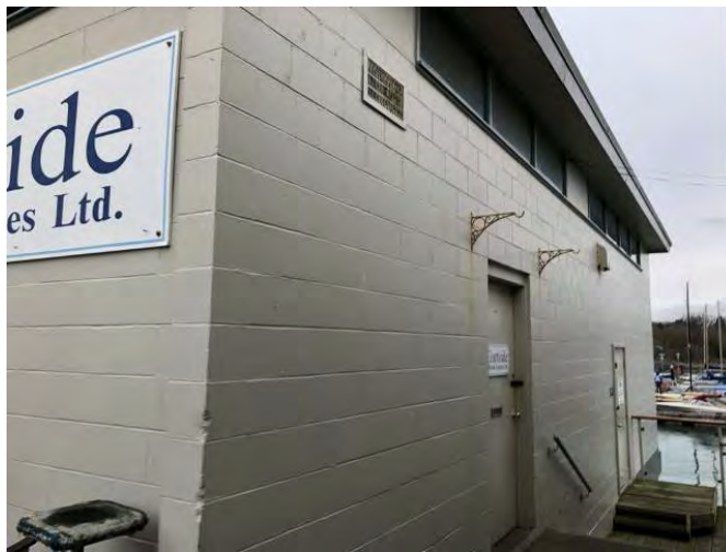
Photo #38: Dockworks North Elevation.
