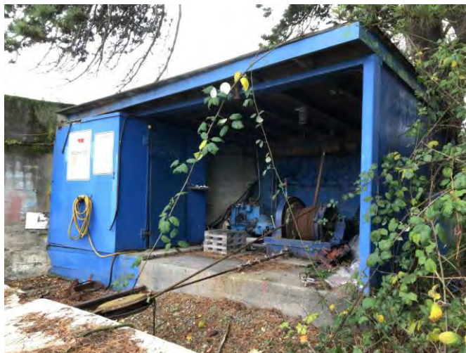
Photo #54: Marina Way Building.
