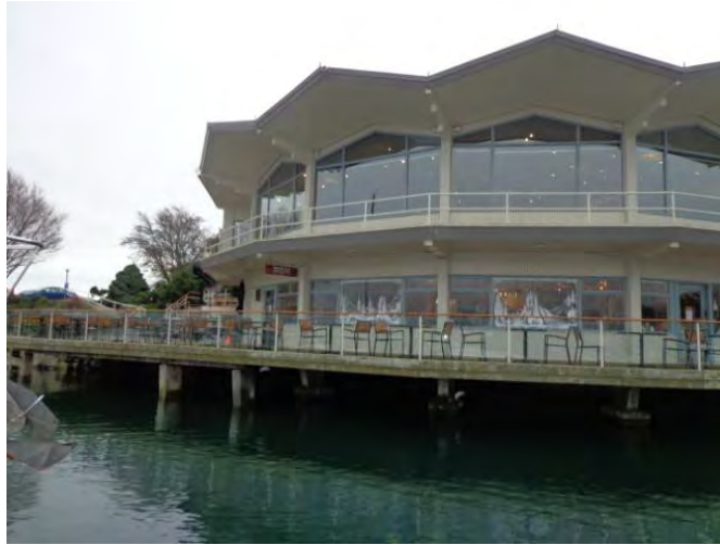
Photo #1: Restaurant North Elevation
