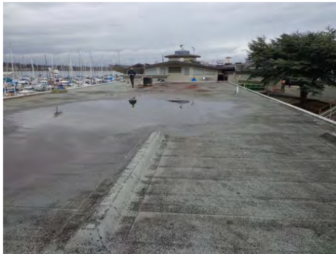
Photo #32: Office Roof Looking North
