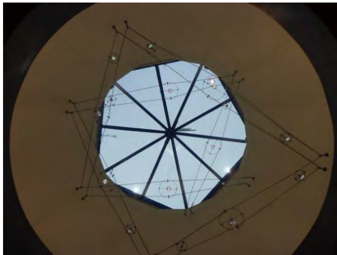
Photo #9: Restaurant Skylight
