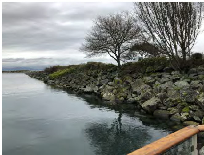
Photo #69: Breakwater - Typical.
