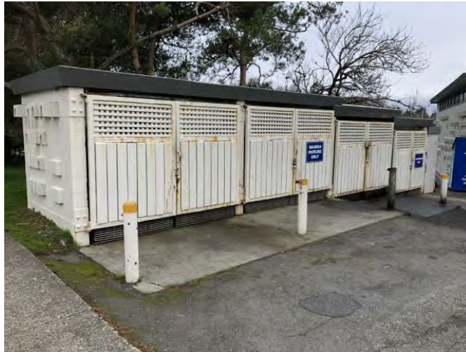
Photo #76: Garbage Enclosure.
