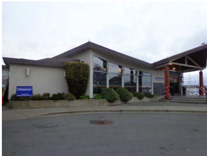
Photo #2: Restaurant East Elevation
