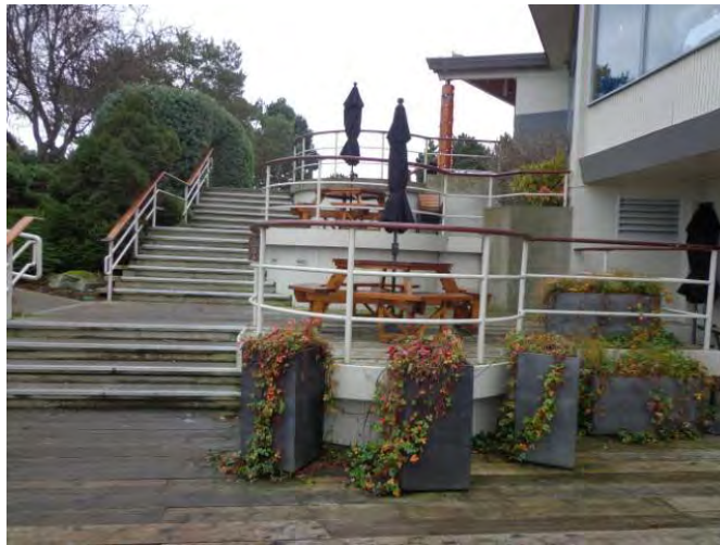
Photo #14: Restaurant Staircases and Railings - Typical
