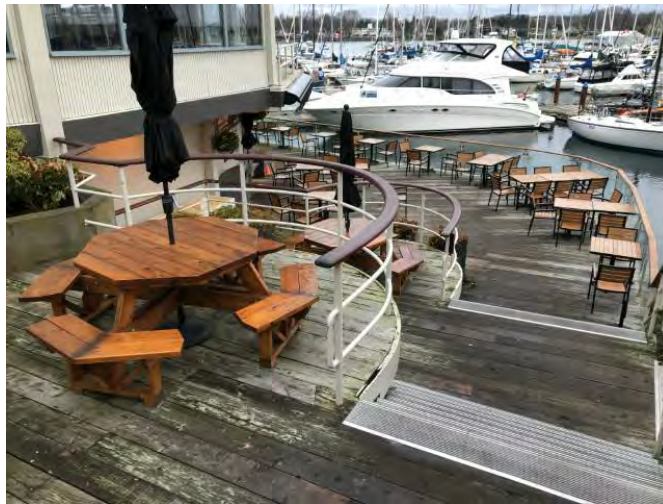
Photo #13: Restaurant Wood-framed Exterior Deck.
