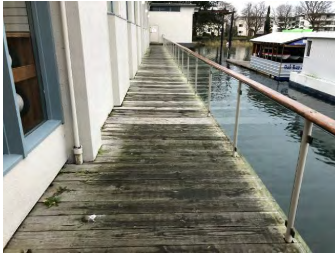
Photo #58: Wood-framed Walkway with Railing - Typical.
