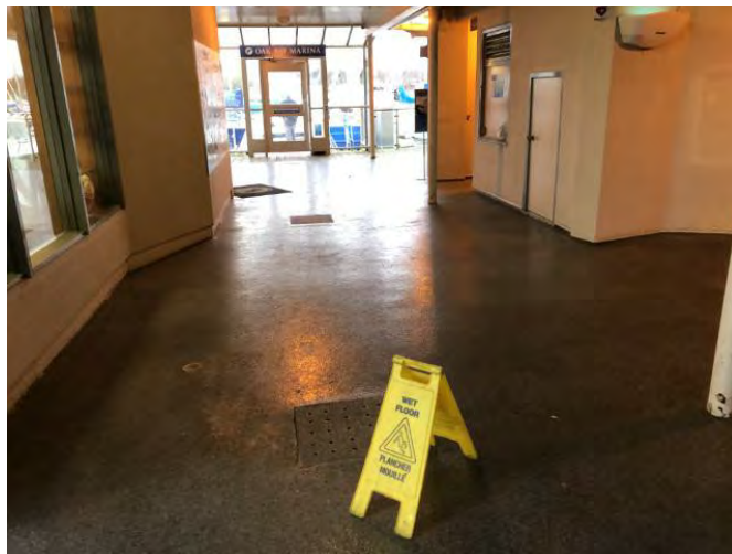
Photo #57: Covered Walkway.
