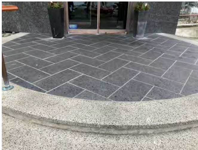
Photo #15: Restaurant Entrance Pavers.
