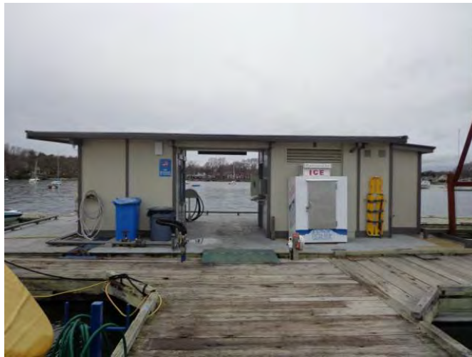
Photo #50: Marina Dock Gas Pump Station
