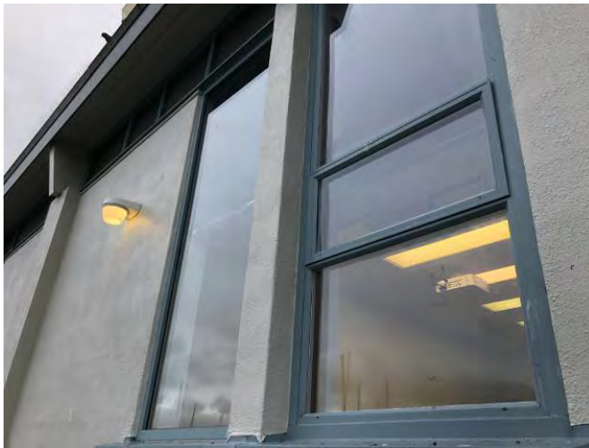
Photo #30: Office Walls and Windows - Typical.
