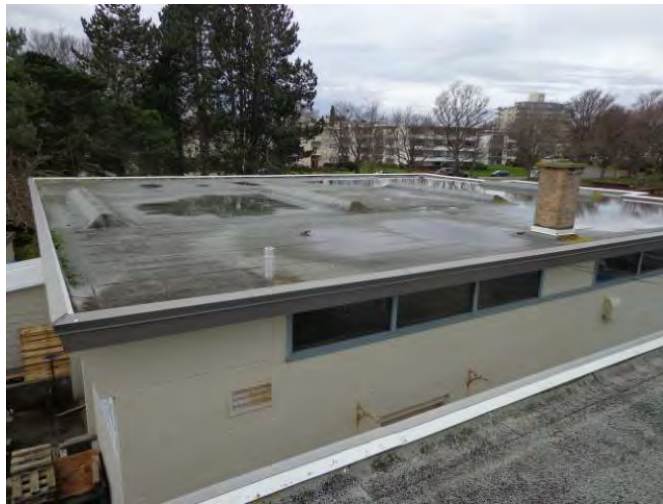
Photo #43: Dockworks Roof
