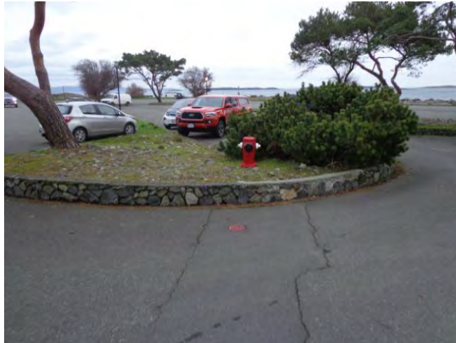
Photo #70: Site Fire Hydrant
