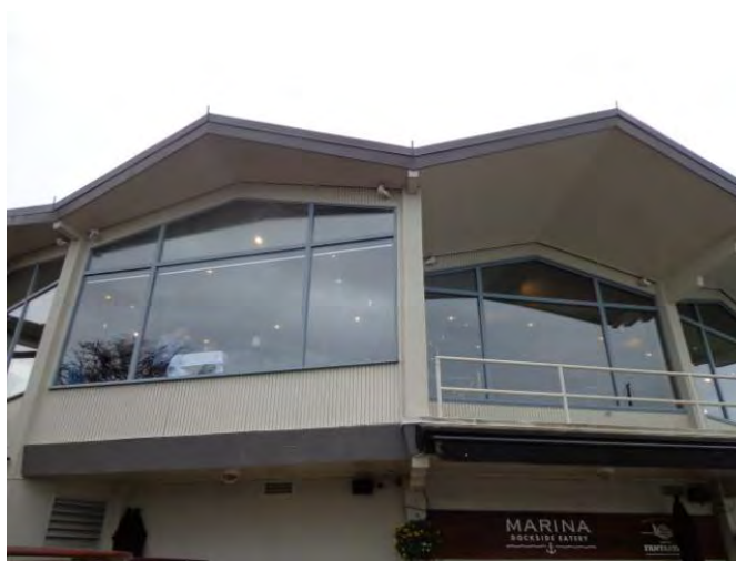
Photo #6: Restaurant Walls and Windows - Typical
