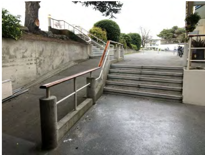
Photo #56: Site Walkways and Staircases - Typical.
