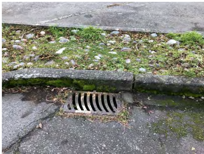
Photo #60: Parking Lot Catch Basin - Typical.
