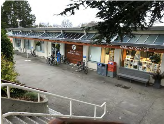
Photo #28: Office East Elevation.
