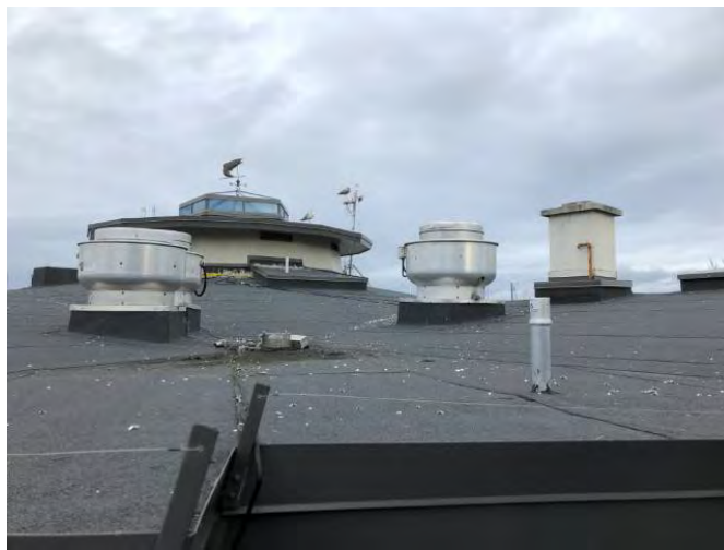
Photo #8: Restaurant Roof - Typical.
