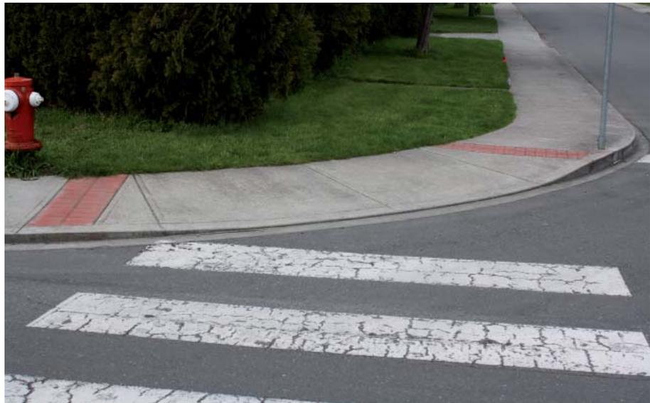
*Example of recent curb ramp improvements in Oak Bay aimed at ensuring an appropriate slope and tactile warning strips that identify the crossing point.*
