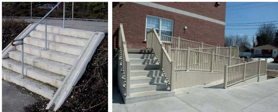
*A bicycle stairway channel (left) and wheelchair accessible ramps (right) are examples of features that can be built into staircases to better accommodate bicycle and wheelchairs.*
