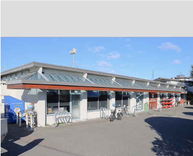
Building 2 - Marina Sales & Service
